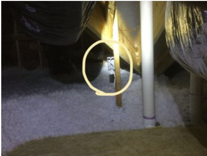
Open Junction Boxes in the Attic.
